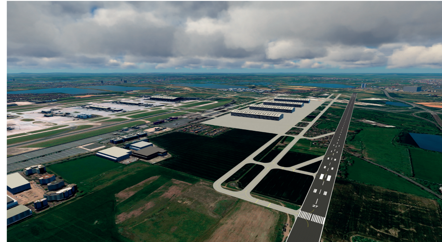
Rapid Prototyping in Action: A reconstructed Heathrow Airport starts to take shape.
